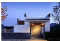
Household Energy Storage
