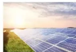
Energy Storage System
